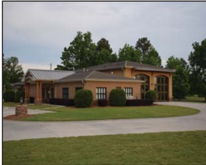
Pelham Batesville Fire Station #3
