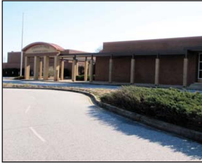
Chandler Creek Elementary School
